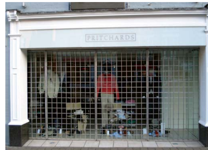
This grille is set behind pilasters and is removable
