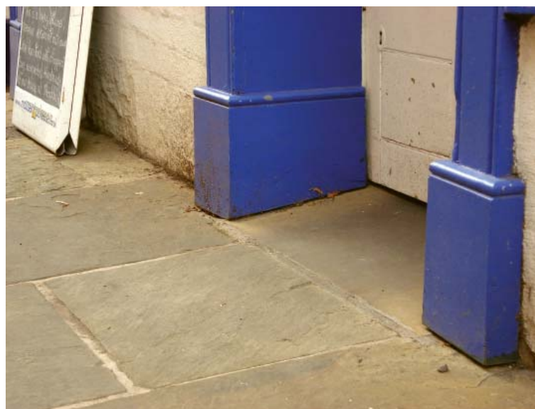
Pavement ramped slightly to ease access into the shop door
