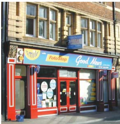
Posters, lettering and colour spoil the appearance of this shop front, and the wider street
