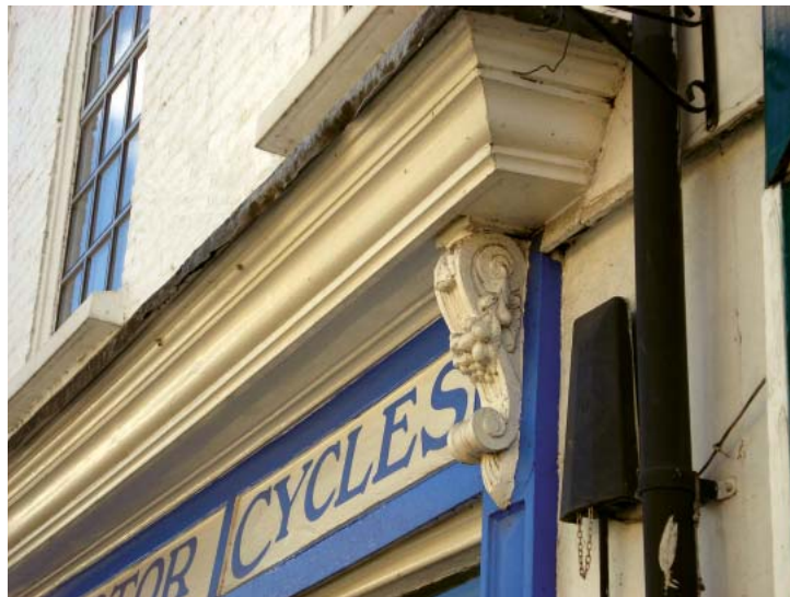
Projecting cornice and brackets give depth to the façade
